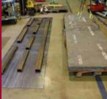
2. Put plate supports on top (in this case, U-beams)
