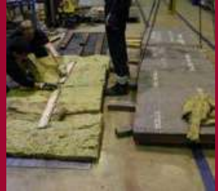
3. Cover it with insulation
